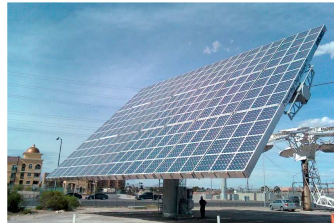
This impressive two - axis tracker in Las Vegas, USA, supports multiple point - focus concentrator modules solar cells and is rated at 53 kW 23 .
