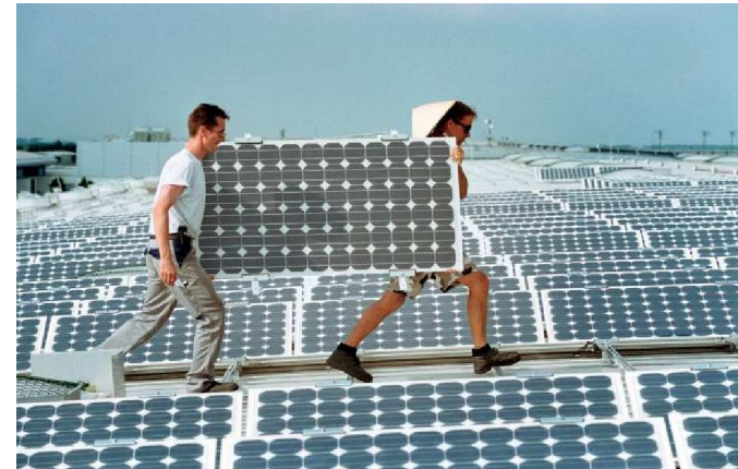
Each of these PV modules contains 72 monocrystalline silicon solar cells 21 .
