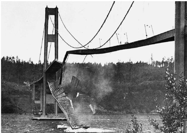
Tacoma Narrows bridge at catastrophic failure
